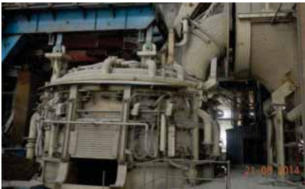
100T EAF, Monnet Ispat & Energy Ltd., Raigarh, India
